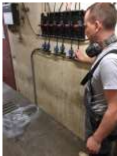
Wash water and disinfection is washed out – cleaning done
